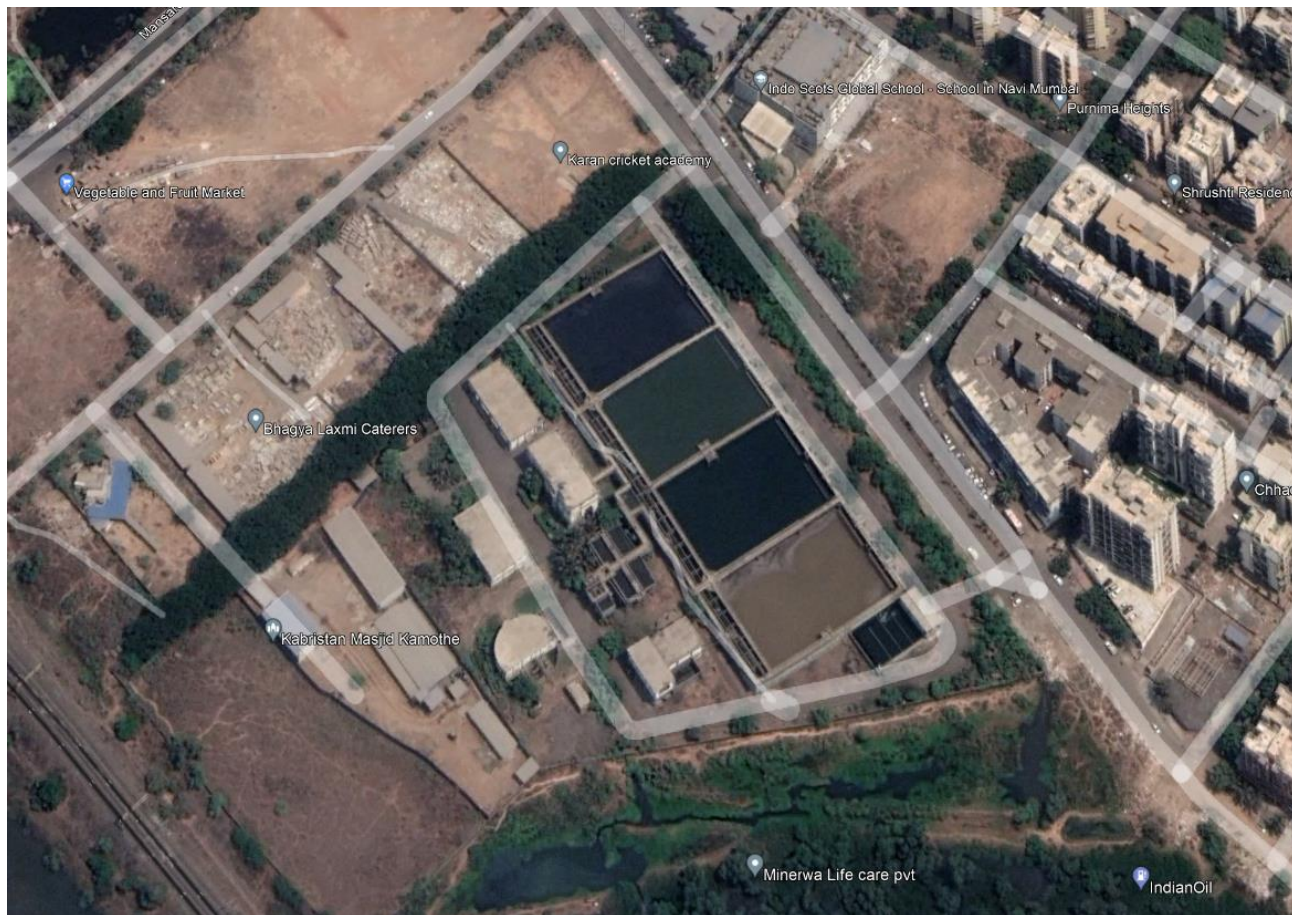
Figure 6.12: Kamothe STP (19° 0'48.62"N 73° 5'13.02"E), Capacity – 85 MLD
