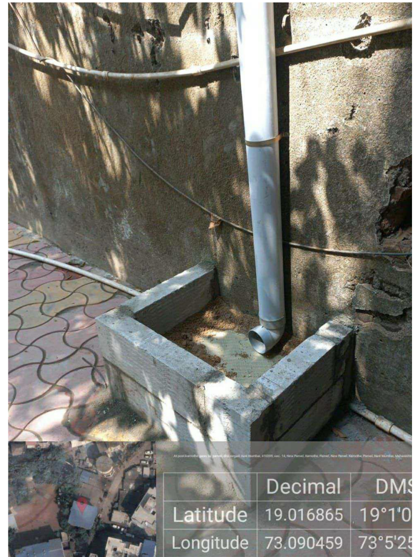
Installation of Rooftop Rainwater Harvesting system in public building
