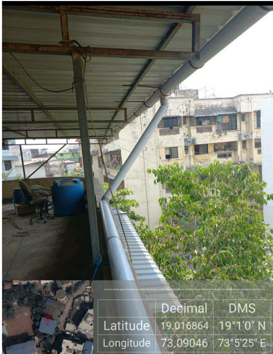
Installation of Rooftop Rainwater Harvesting system in public building
