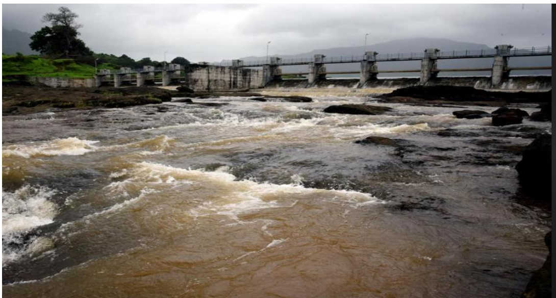
Figure 6.4: Dehrang Dam, Panvel
